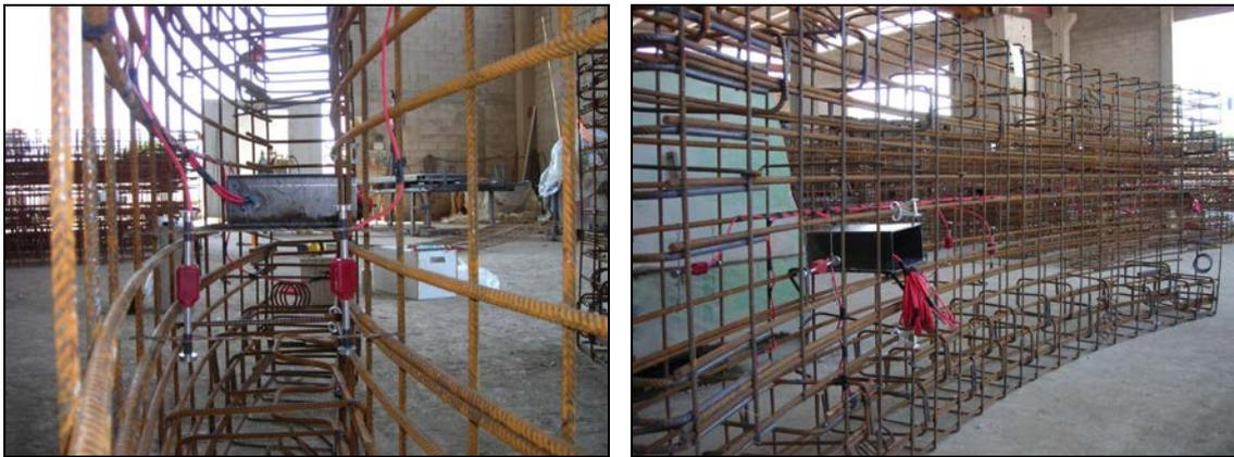
**Figure 6 Vibrating wire strain gauges installed on the steel supporting structures of the final lining segments and steel boxes for the future GENESI nodes housing.**
