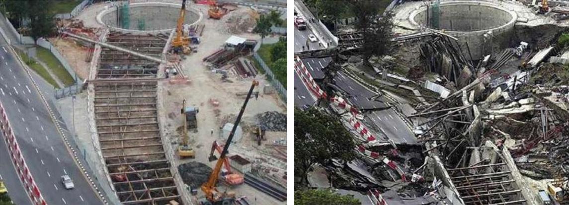
**Figure 2 Singapore MRT Spring 2004 before and after the collapse (images taken from internet “The Code of Practice for Risk Management of Tunnel Works ITA Conference Seoul, April 25, 2006”).**
