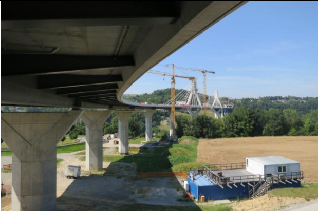
Bridge construction. GENESI system is extended over the complete structure
