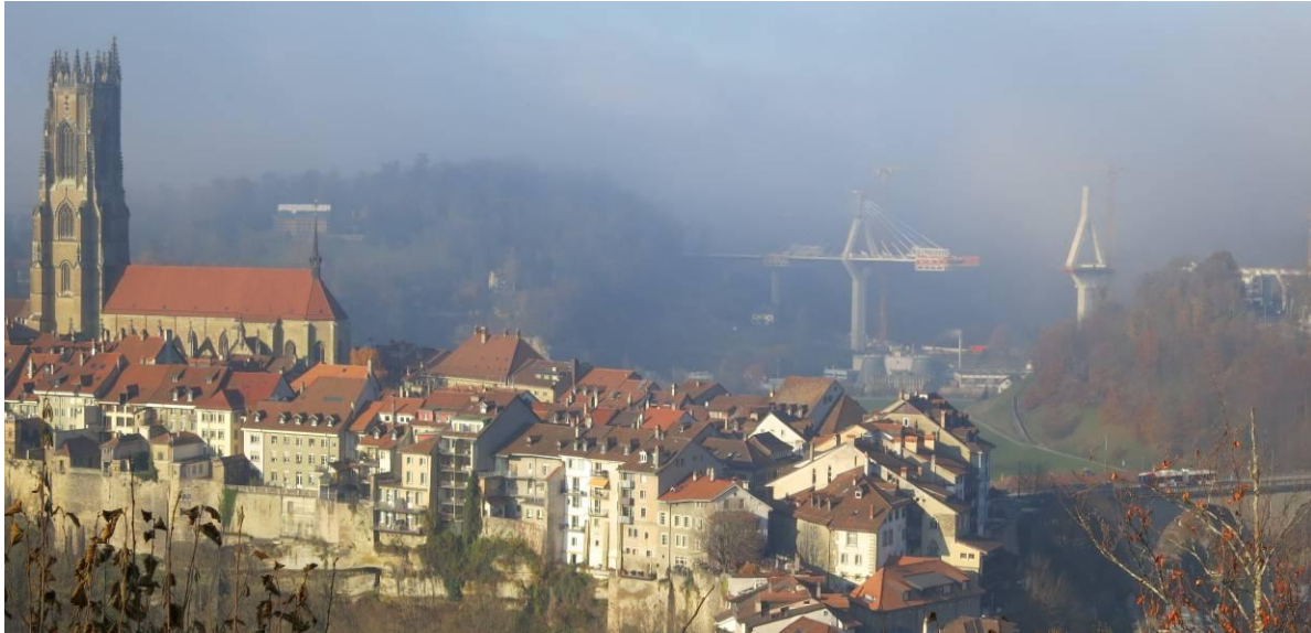
Historic town of Fribourg with the construction site of the Pont de la Poya in the background
